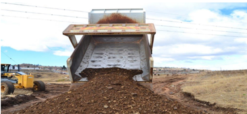
3. Dumping of road layer uncrushed G6 material
