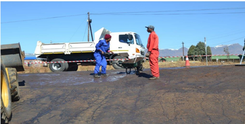
12. Application of the slurry
