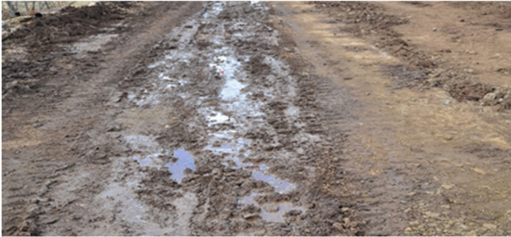
1. The road as it was before treatment
