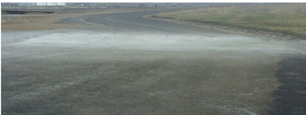
13. Complete soil binder surfaced road
