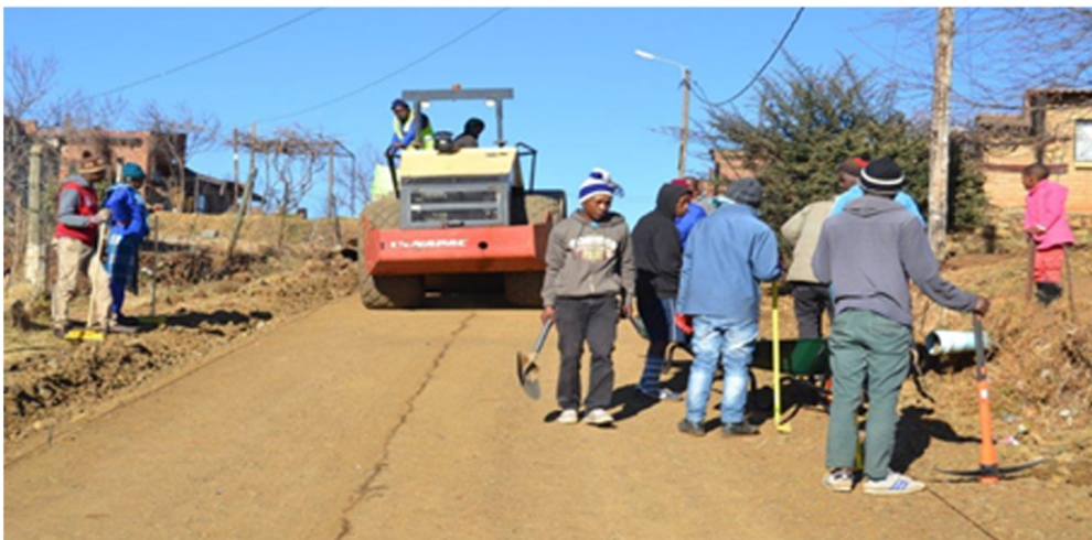
8. Final Compaction (Preparation of the final level)
