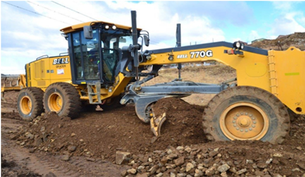
4. Spreading of road layer uncrushed G6 Material
