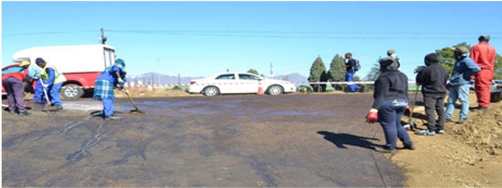
10. Application of Black Top Asphalt (BTA) bitumen
