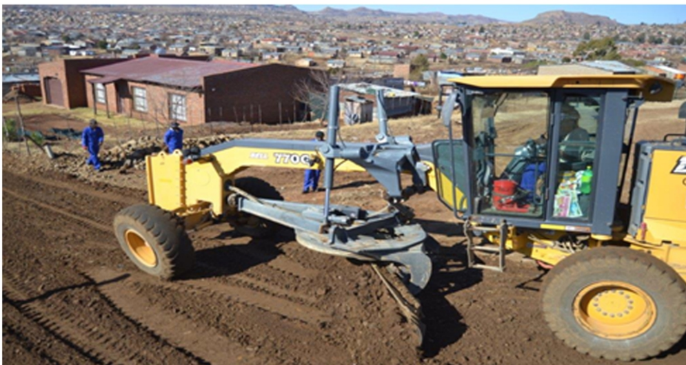
6. Mixing of crushed G6 road laying material with soil binder
