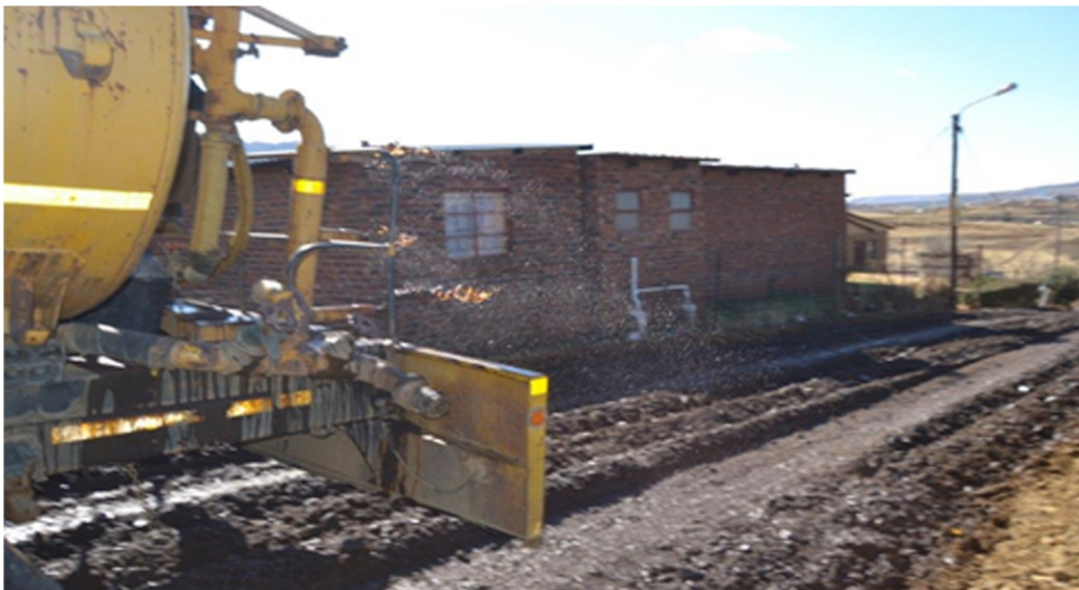
5. Stabilisation by pouring soil binder mix on the road surface
